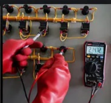
Maintenance of distribution cabinet
